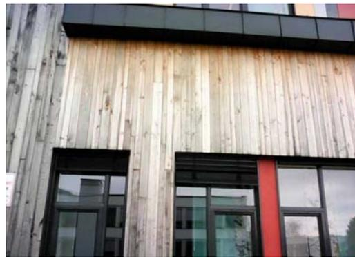
**Figure 4:** Example of not uniform discoloration of the facades due to natural weathering
