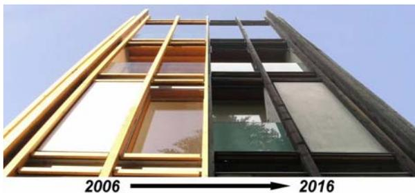
**Figure 1:** Appearance change of the unprotected wooden structure in time
